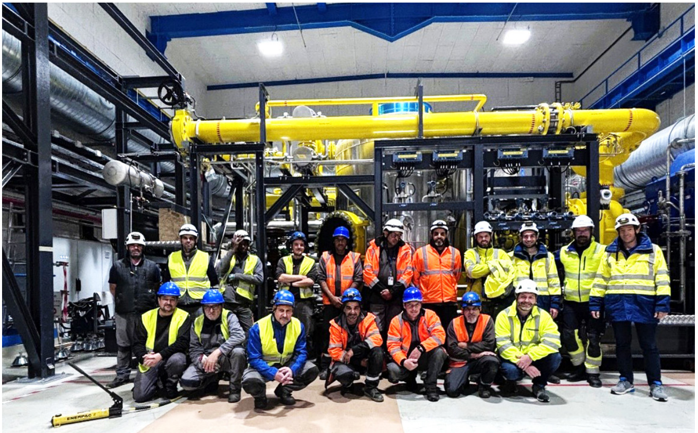
Installation of the compressor stations of the HL-LHC helium liquefiers
