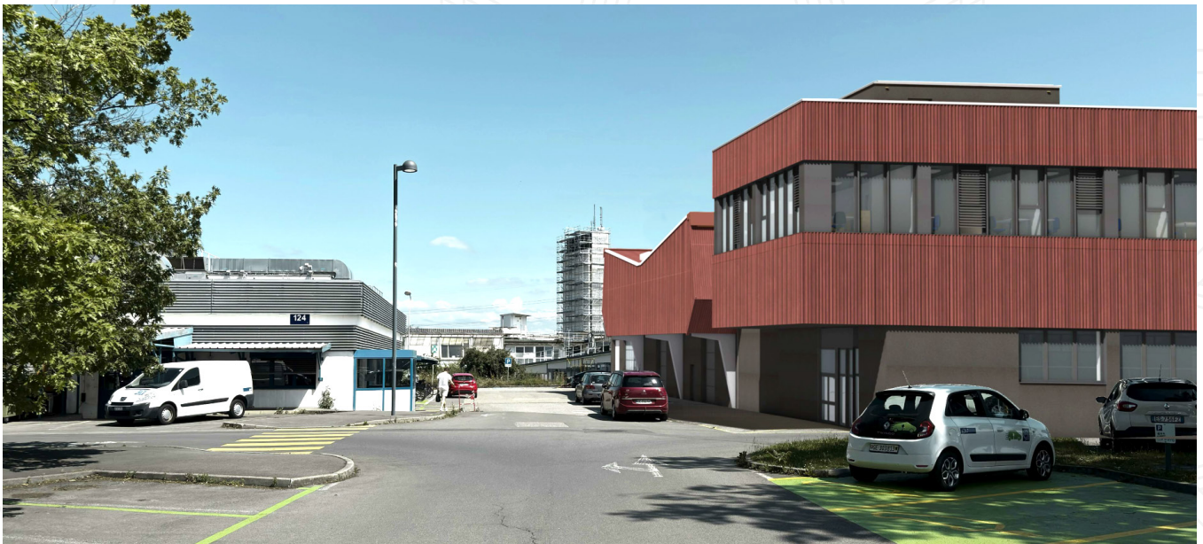
B72 and B100 refurbishment.
