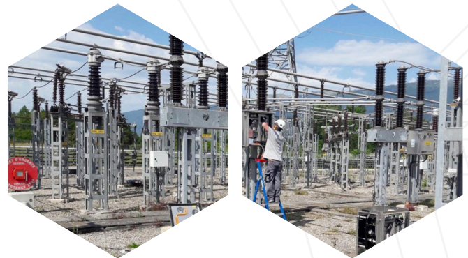
Electrical works on the CERN site
