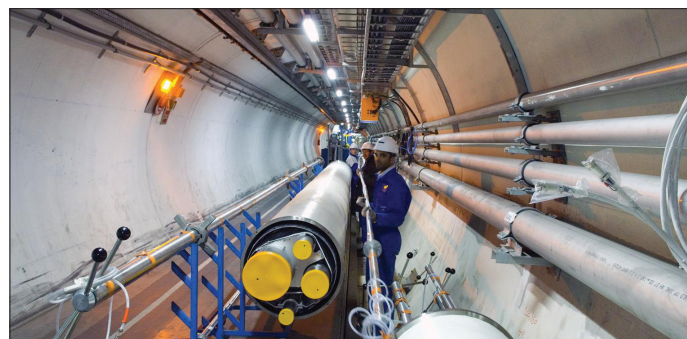
Fig. 3. Installation of the cryogenic distribution line (QRL) in LHC sector 1-2, the last to be equipped, in May 2006. Each sector involved placing 325 elements and carrying out almost 2000 internal welds.
