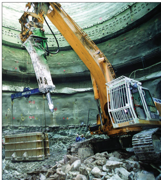
Fig. 1. A number of events occurred during construction that necessitated amendments to the LHC contracts. During construction of the ATLAS caverns and access shafts (left), the design of a vault using reinforced concrete beams was found to be technically unacceptable and had to be replaced. During excavation at the CMS site (right), meanwhile, the discovery of unforeseeable ground conditions required significant changes to the approach and led to the submission of disputes to an adjudication panel. In all cases, they were successfully resolved.
